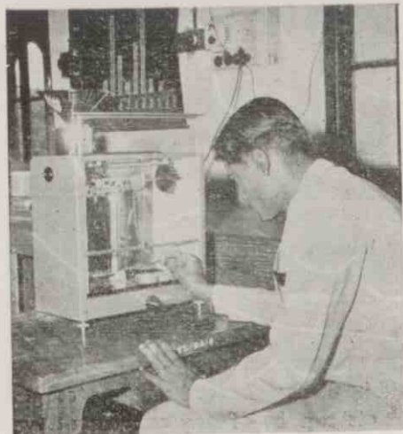
FIG. 48—The chain-o-matic balance will weigh accurately to 4 decimal places.
